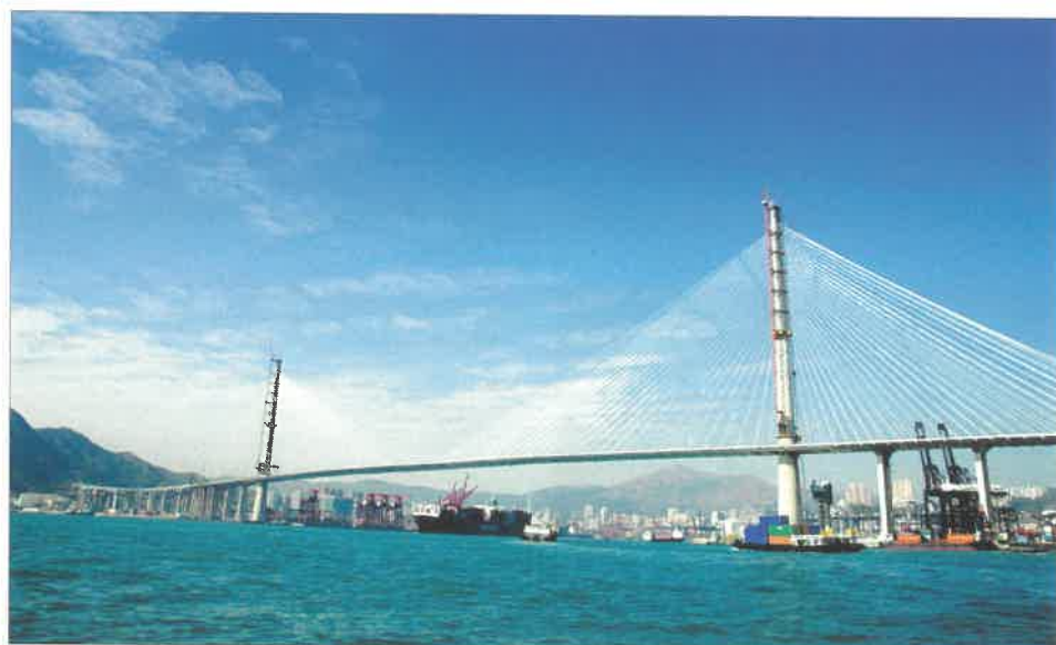
23. ábra. Stonecutter Bridge – Hongkong; nappal
