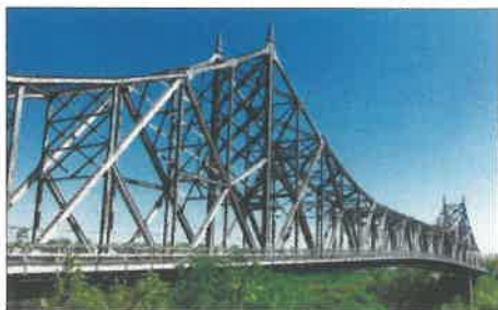
2. Massena Bridge – New York
