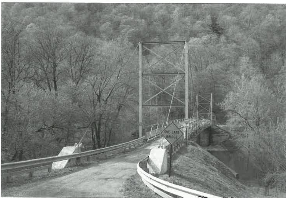
9. Corbin Bridge – Pennsylvania, USA
