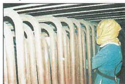
The life time of superheated tubes can be extended many times by using TE-6, TE-7 and TE-22 coatings. The TE-6 and TE-7 coatings are patented by Telatek.
